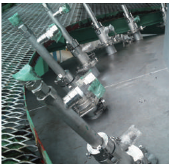
Nozzle installation locations in a cooling tower
